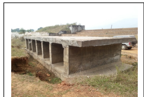
Photograph of incomplete culvert on road from Dimapur to Kujuni of Gosani Block under Gajapati District
